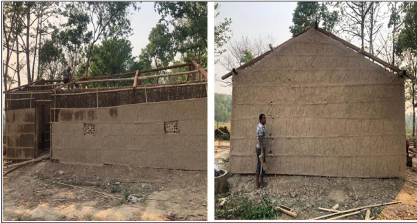
Fig 1: The Deukhuriya house which is currently being constructed (Source: field survey)
